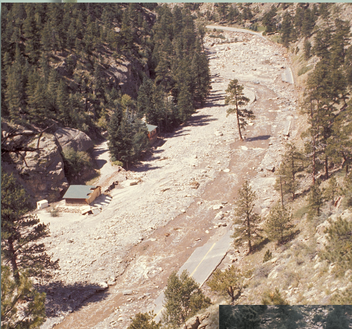
Figure 7 (Above). Upstream view of the Big Thompson River showing extreme flood damage to U.S. Highway 34 upstream from Drake. The U.S. Geological Survey estimated the flood's peak discharge to be 28,200 cubic feet per second in this area.
