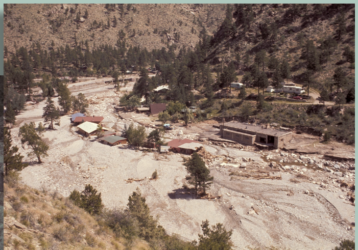
Figure 5 (Above). Damaged and destroyed homes and extensive flood-deposited sediment along the Big Thompson River. This photograph was taken from the hillside looking downstream at Drake. River flow is from bottom right to top center.
