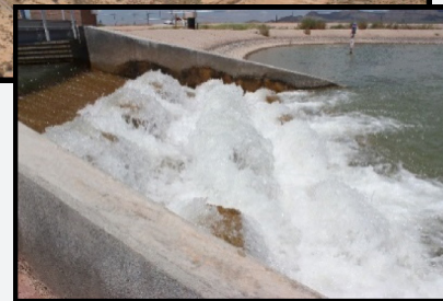
BASIN INLET STRUCTURE
