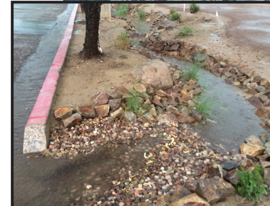
CURB CUT AT ROADWAY EDGE
