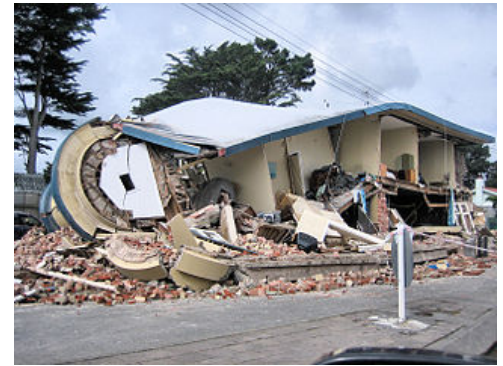
Building damaged in 2011 Christchurch earthquake. Wikipedia, Martin Luff
